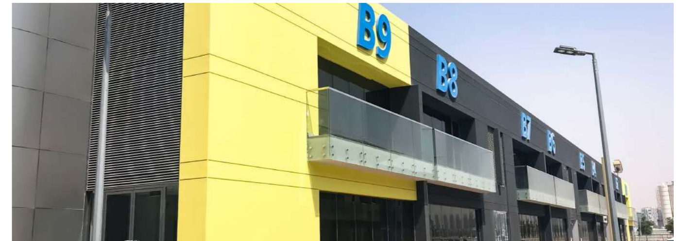
Procom Middle East Offices and Warehouses - Dubai Silicon Oasis
